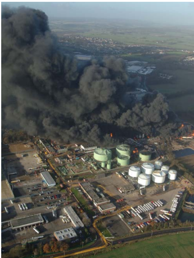
Figure 1: Buncefield oil storage depot, Hertfordshire (photo courtesy Chiltern Air Support Unit)
